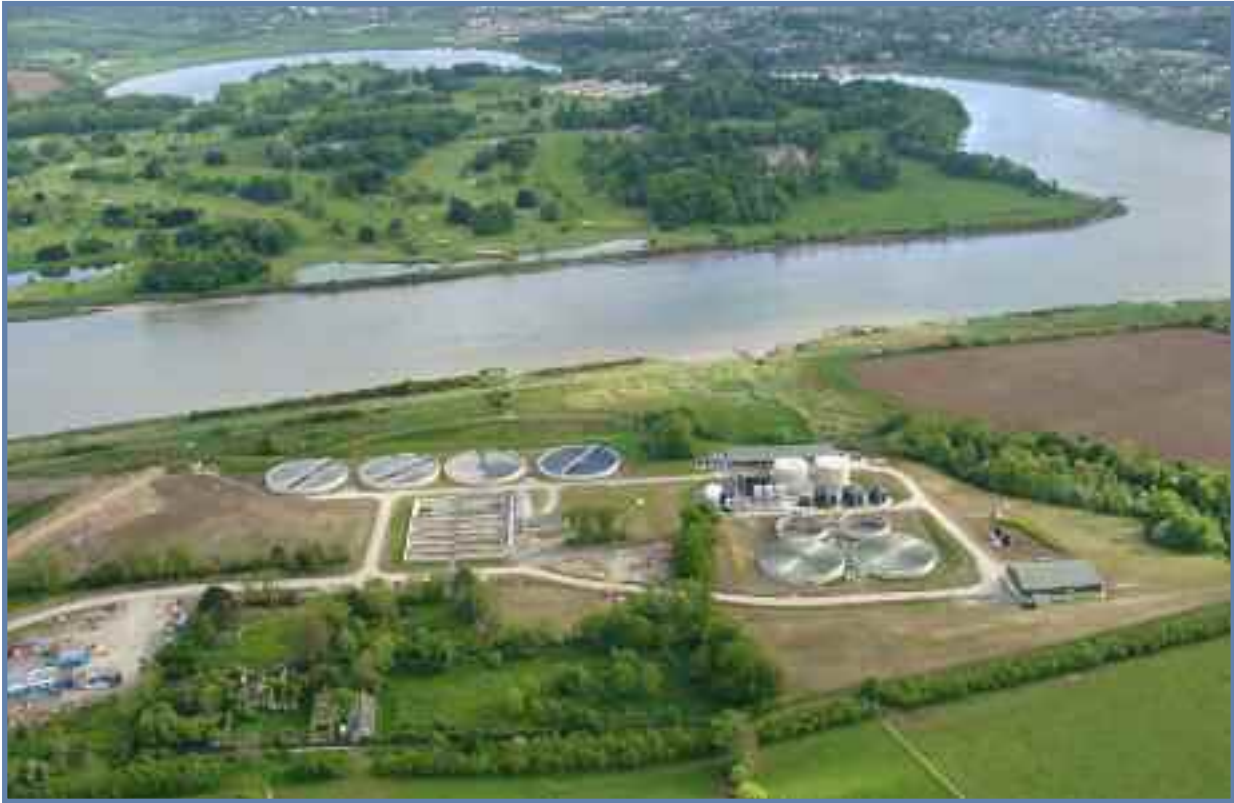
Waterford City Wastewater Treatment Plant
