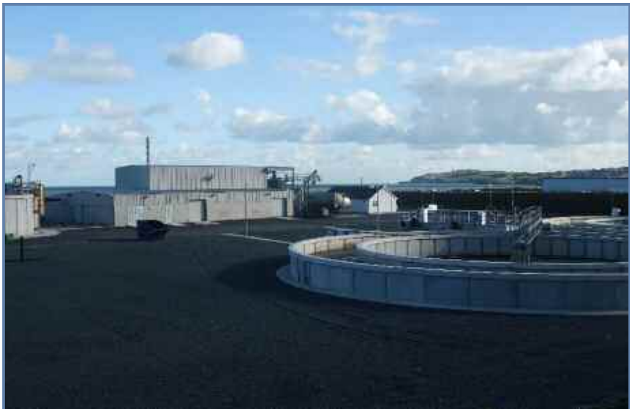
Wicklow Wastewater Treatment Plant
